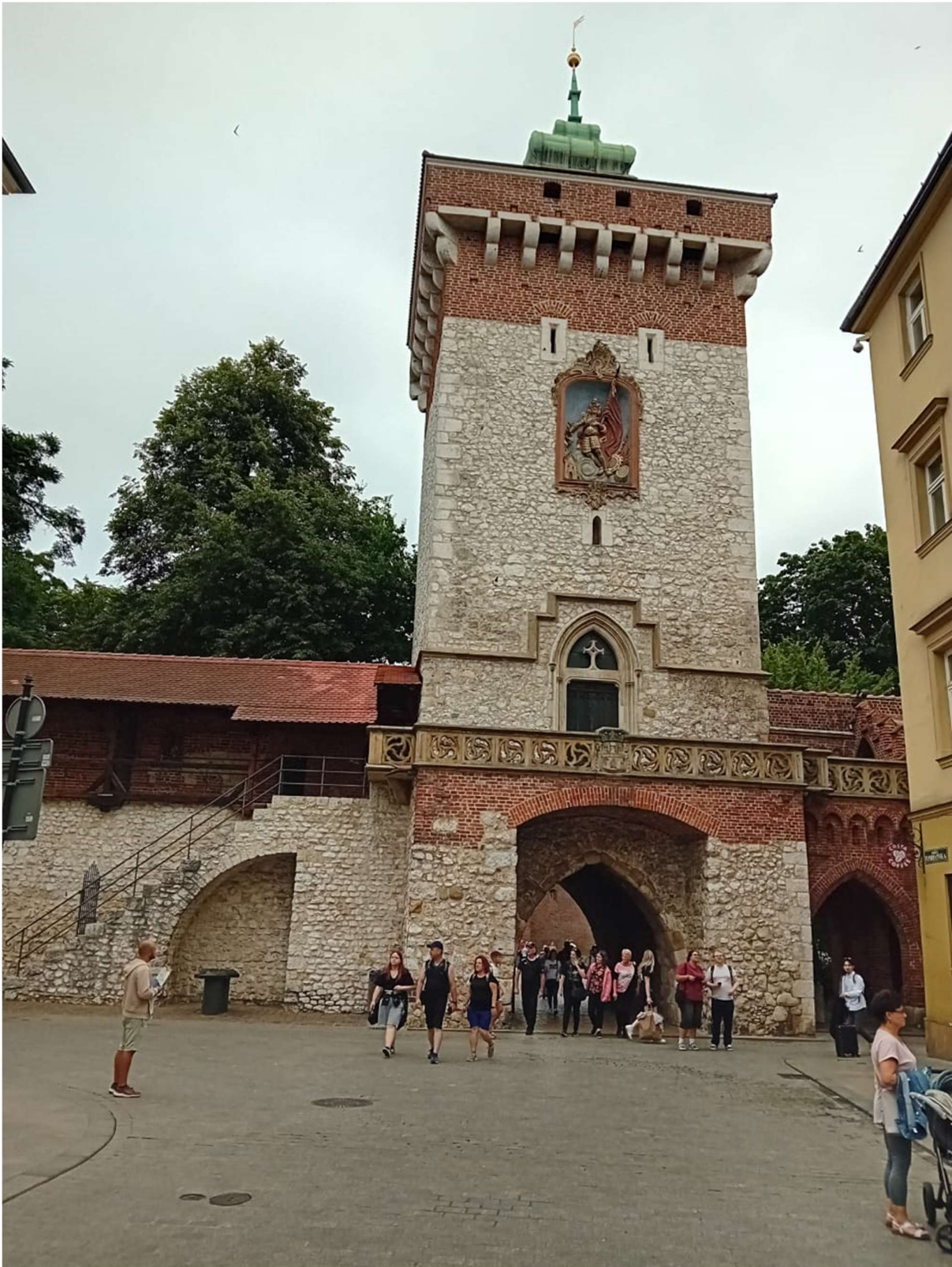
Figure 2: Gate on the City Walls
