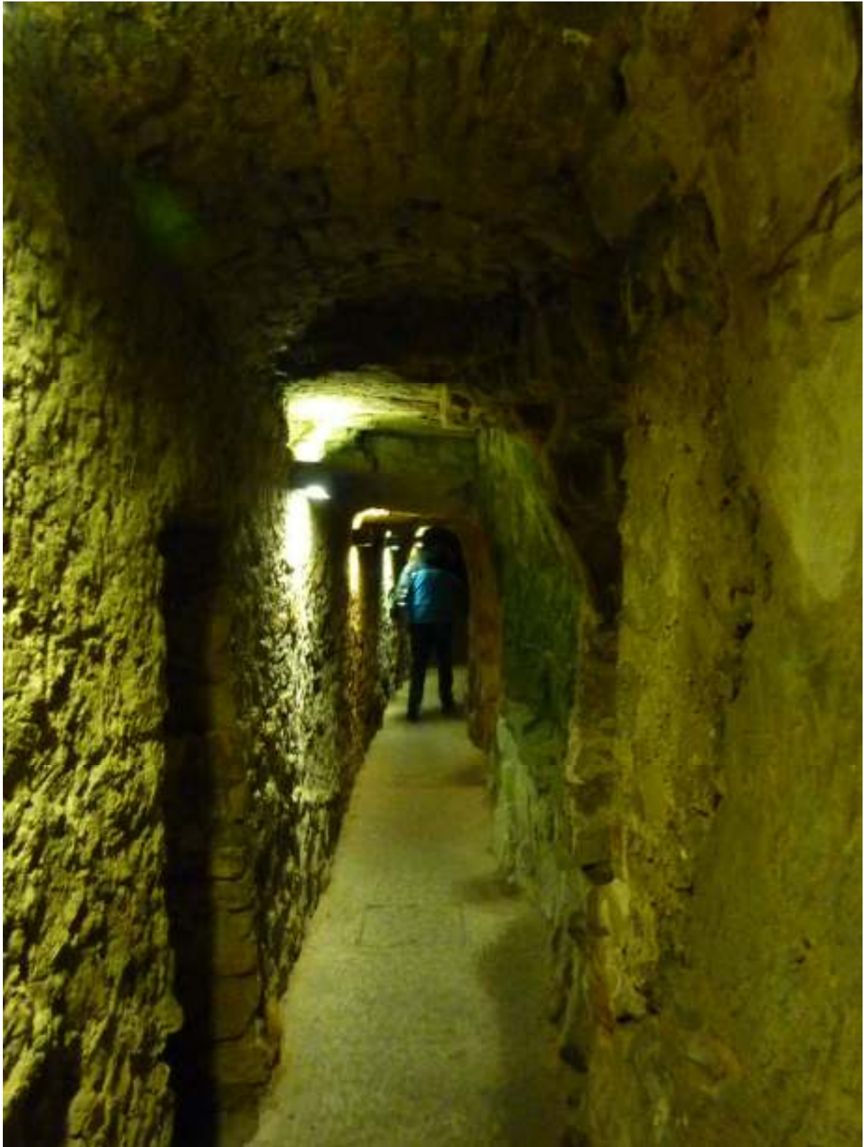
Inside the Casements (Gun fortifications built into cliffs). A labyrinth of tunnels, and tight spiral staircases.
